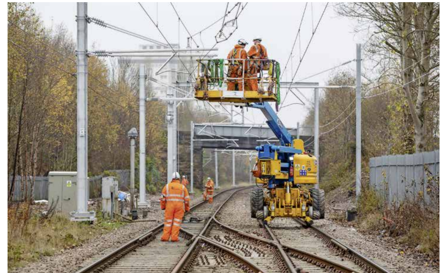
Carillion carries out work on electrification of Scotland’s Whifflet Line. Carillion’s collapse last year is indicative of the type of problems encountered by bidding for contracts at low margins, requiring revenue growth that does not materialise. CARILLION.
