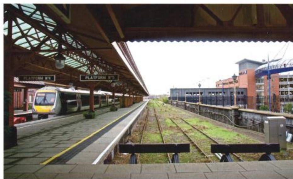
Moor Street: the Midlands Rail Hub project would see platform 5 brought back into use, plus a new platform 6 built on the right hand side here. JOHN WHITEHOUSE
