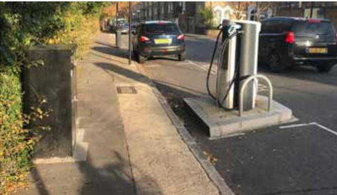
An e-vehicle rapid charge unit located in the carriageway - but note that there will always still be a feeder pillar on the footway.
