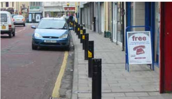
Bollards preventing occasional footway parking, but permanently reducing the usable footway width. With added A-board clutter.
